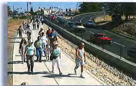
SR 44 Dana to Downtown Opening, October 2010
