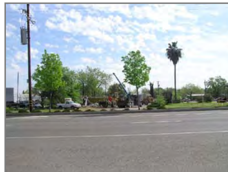
El Rancho Motel during demolition
