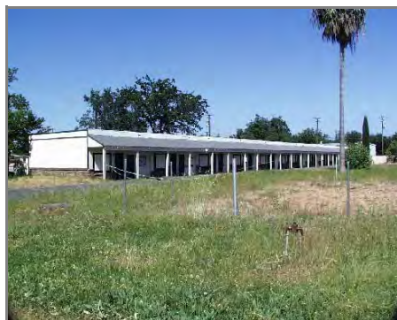
El Rancho Motel before demolition Photos courtesy City of Redding
