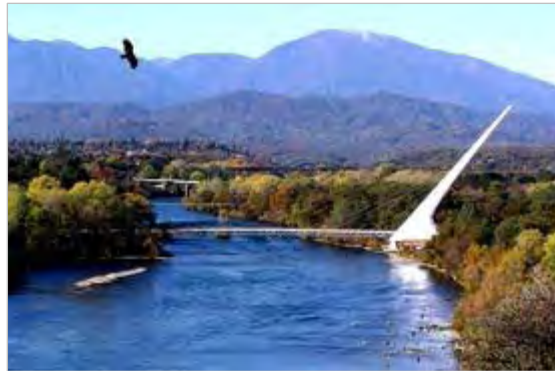
The Sundial Bridge: A community landmark and part of Shasta County's growing bicycle and pedestrian infrastructure
