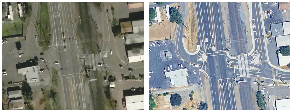
SR 273 and Girvan Road intersection in 2020 (left) and in 2024 (right). Image source: Google earth 2020 and 2024.
