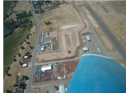
Fall River Mills Airport Runway Expansion
