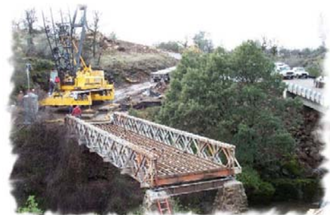
Bridge Replacement-Wildcat Road
