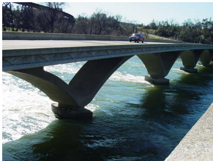
Figure 30 - Benton Drive over Sacramento River
