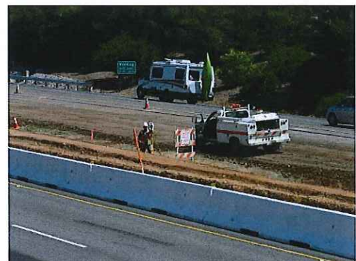
South Redding Six-Lane Construction, 2011.
