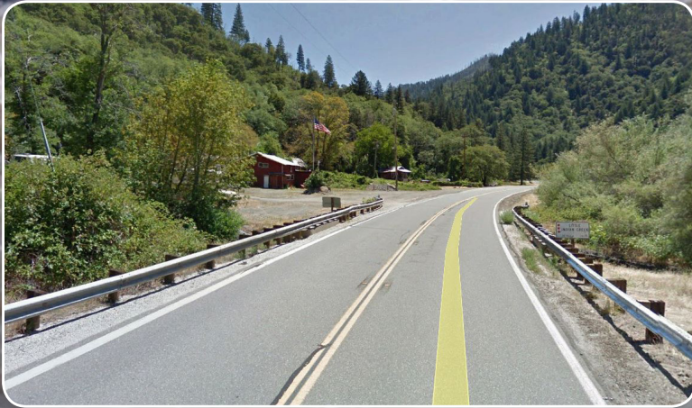
ROUTE 70 IN PLUMAS COUNTY BEFORE FLOODING
