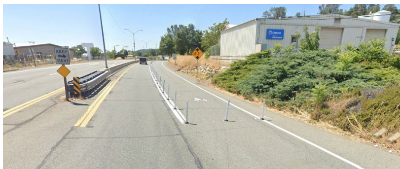
Start of Pilot Class IV Bikeway on Southbound SR 273. Image source: Google, 2023.
