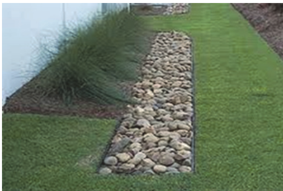
Infiltration and Soakage Trench
