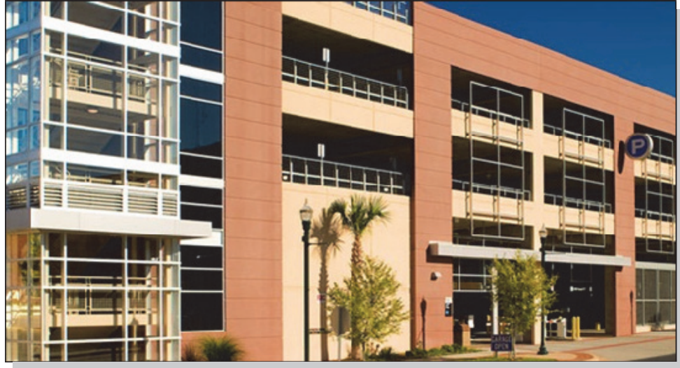
Figure H3 – Example of a Modern Multi-story Parking Structure Sited on a Smaller Footprint
