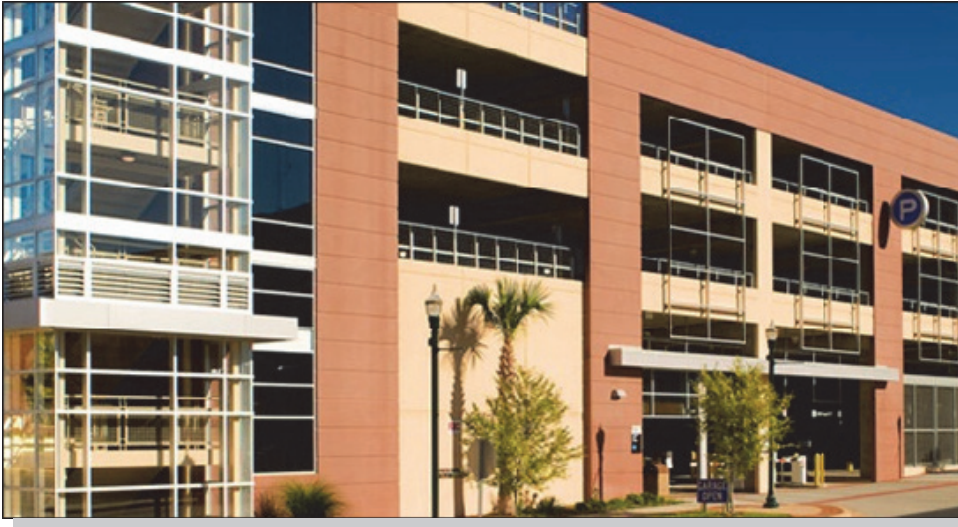
Figure 4 – Example of a Modern Multi-story Parking Structure Sited on a Smaller Footprint
