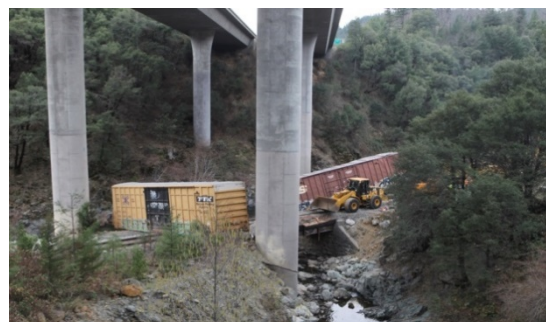
Figure 2 Union Pacific Train Derailment at I-5 in Shasta County, 2014.
