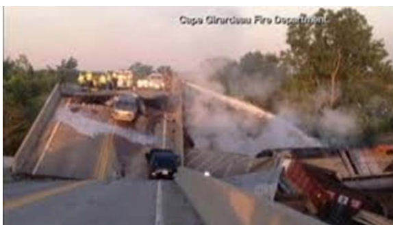
Figure 1 Union Pacific train derailment highway structure collapse, Missouri, 2013.
