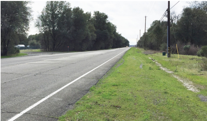
Figure 3.14. Existing Airport Road. Source: Kittleson & Associates, Inc.
