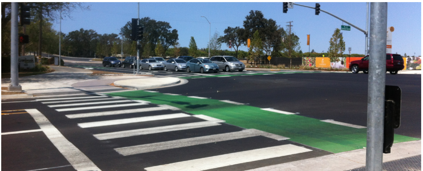
Figure 3.8. High visibility crossings for bicyclists and pedestrians in Davis, CA. Source: Kittelson & Associates, Inc.
