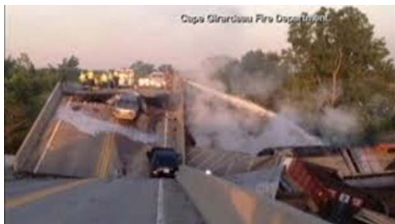
Figure 4 Union Pacific train derailment highway bridge collapse, Missouri, 2013.
