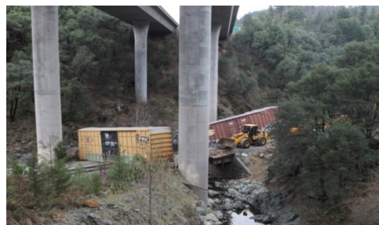
Figure 5 Union Pacific Train Derailment at I-5 in Shasta County, 2014.
