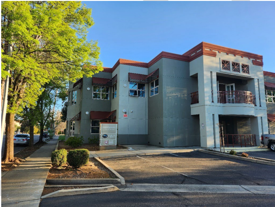
Figure 2: Office of the Shasta Regional Transportation Agency
