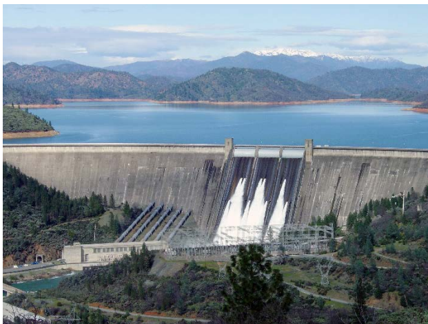
Figure 90. Shasta Dam and the Keswick Dam downstream power the region and protect downstream communities from flooding. Key regional agencies do not know how a dam failure would affect communities and infrastructure. Source: USBR 2021.
