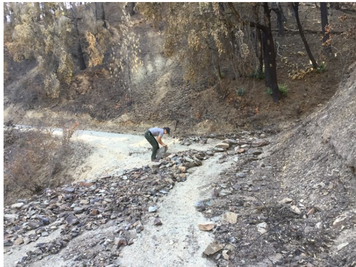
Figure 91. Following the Carr Fire, accelerated erosion of burned slopes on Shasta Bally began depositing large amounts of debris on Mill Creek Road in the Whiskeytown National Recreation Area. Source: NPS 2021.
