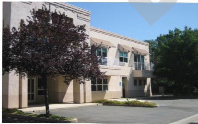
SRTA Offices at 1255 East Street in Redding
