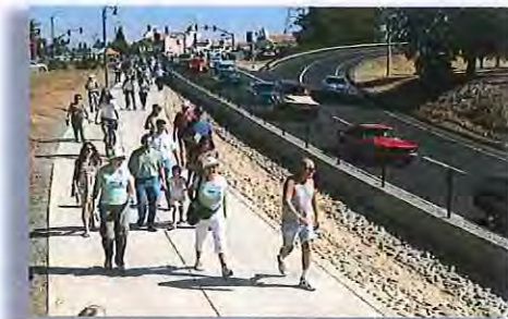
SR 44 Dana to Downtown Opening, October 2010
