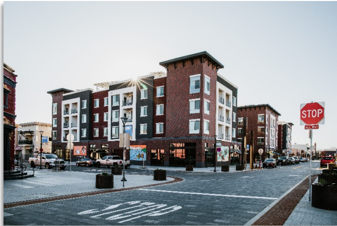
Recently completed Downtown Redding Multi-Use Infill Development Project
