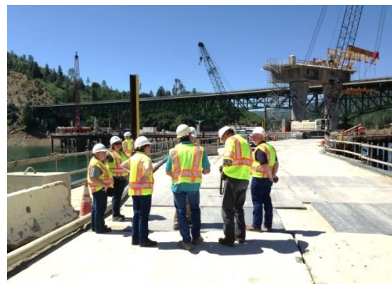
Interstate 5 Antlers Bridge Replacement, June 2013
