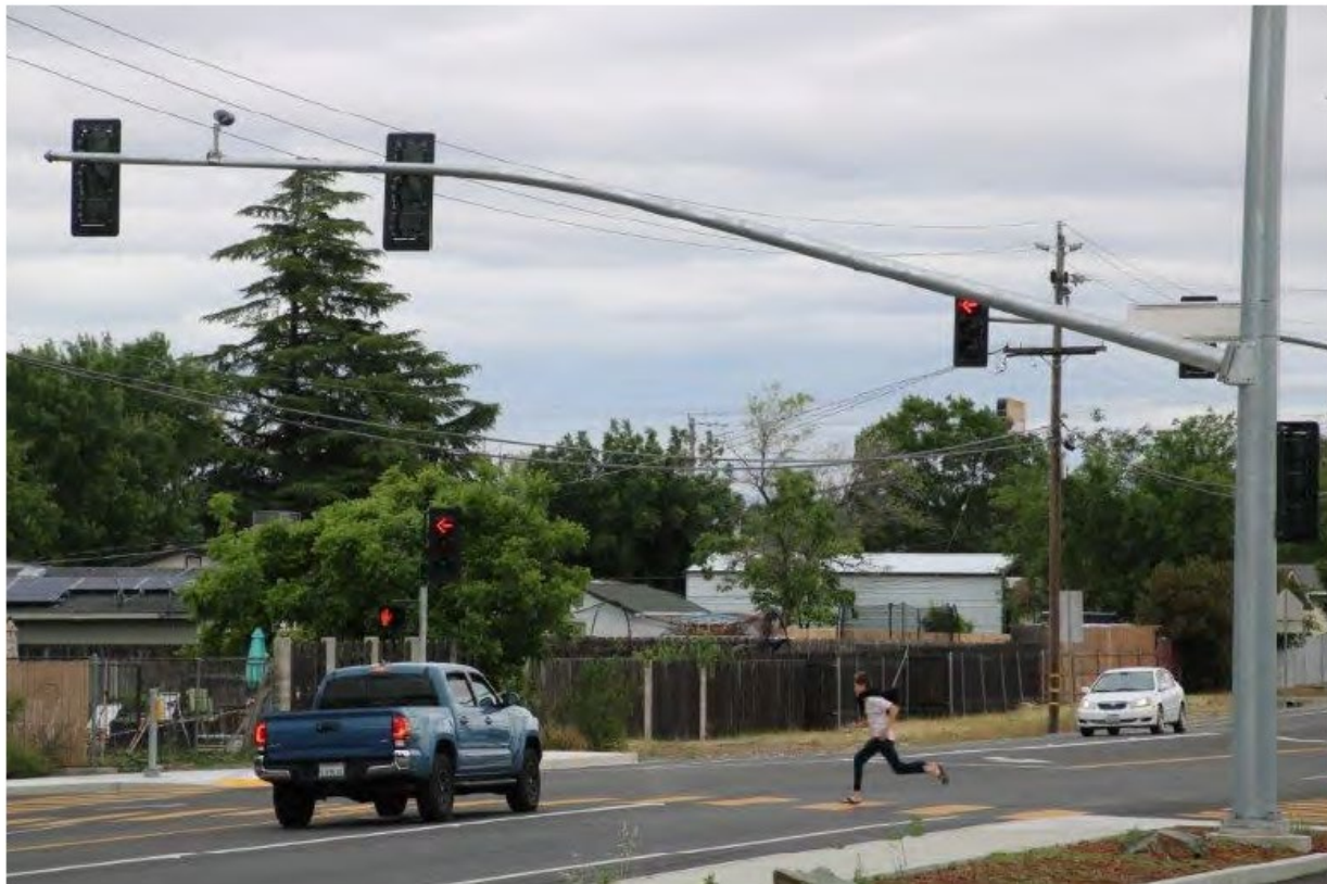
Pedestrian crossing Gas Point Road on recently constructed infrastructure on Gas Point Road
