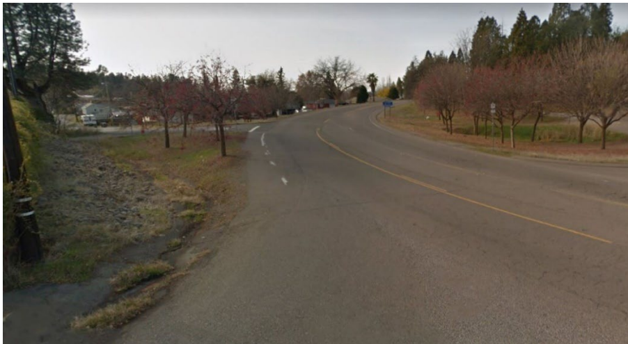
Ashby Rd., on intersection of Ashby Ct., looking South
