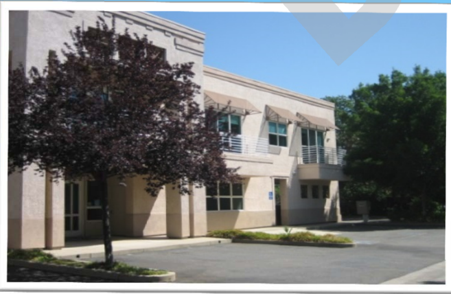
SRTA Offices at 1255 East Street in Redding
