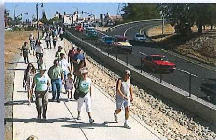
SR 44 Dana to Downtown Opening, October 2010
