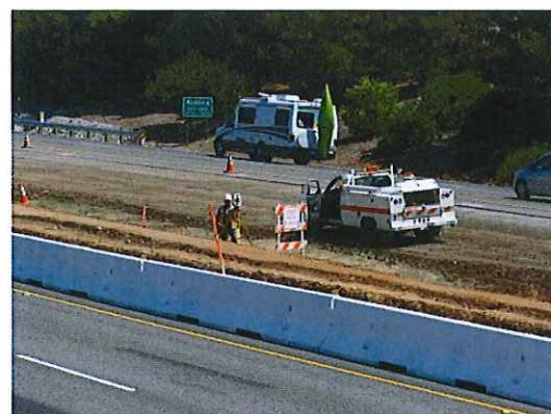
South Redding Six Lane Construction, 2011.
