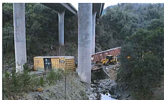
Union Pacific Train Derailment at Interstate 5 in Shasta County, 2014.
