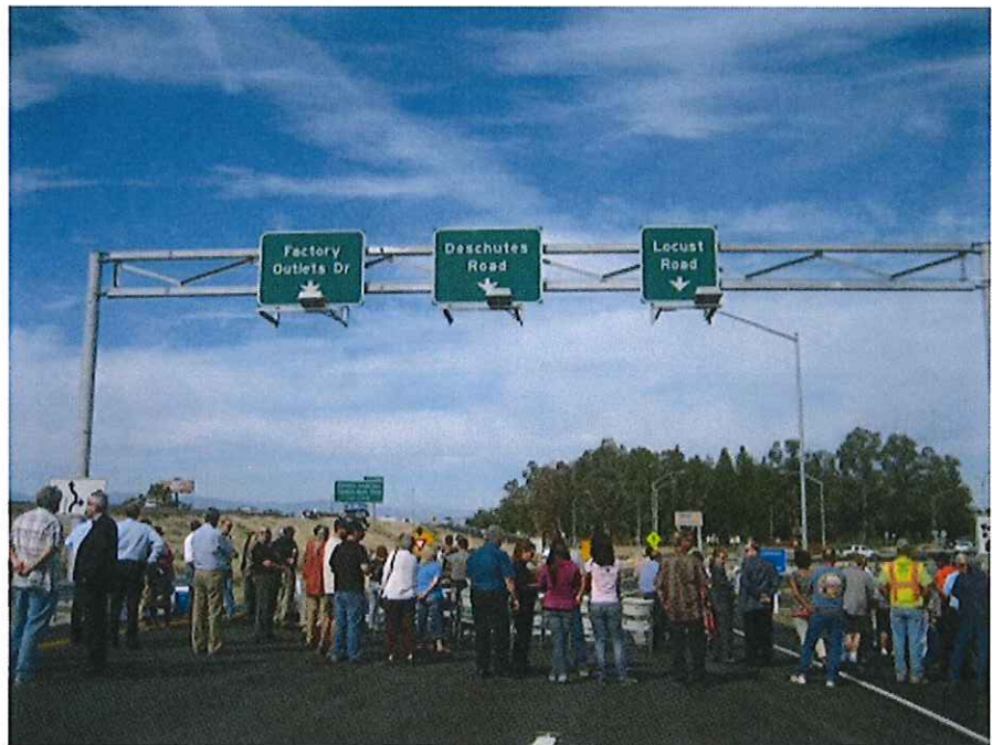
Deschutes Road Interchange Phase 1 Groundbreaking, 2013.
