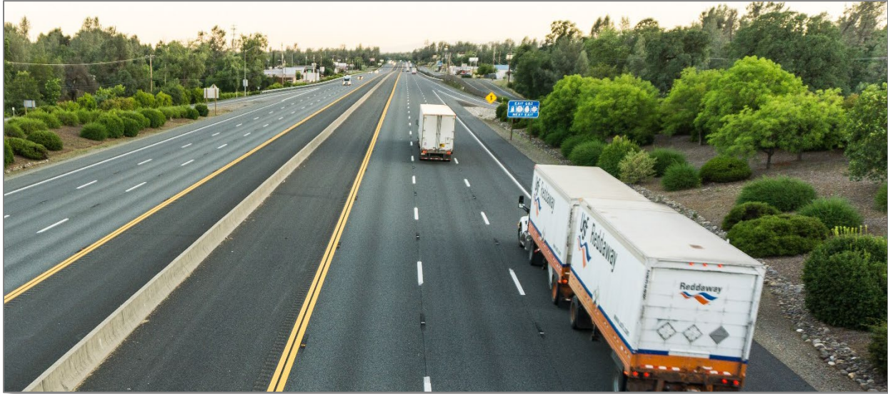
I-5 Looking North in Section I (see attached Project Overview Map)
